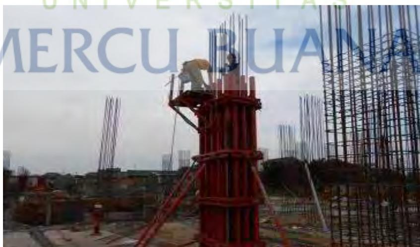
Gambar 5.8 Instalasi Bekisting
