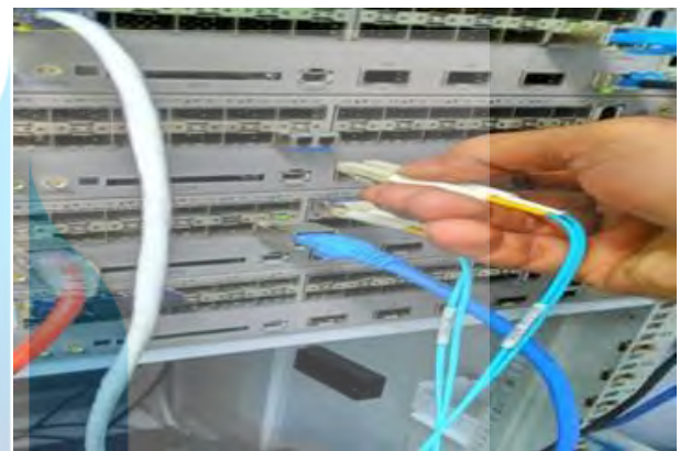
Fig 13: Unplug Fiber Optic Cable on Device Interfaces
