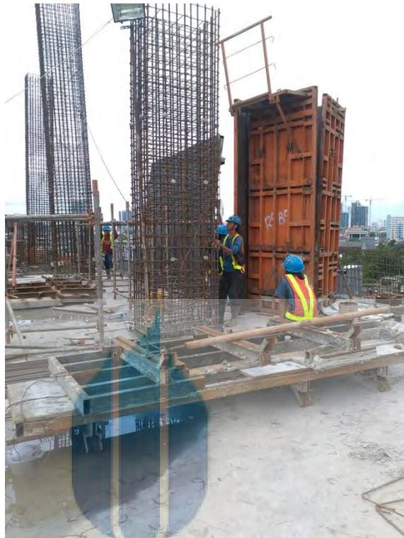
Gambar 4.6 Bekisting Kolom
