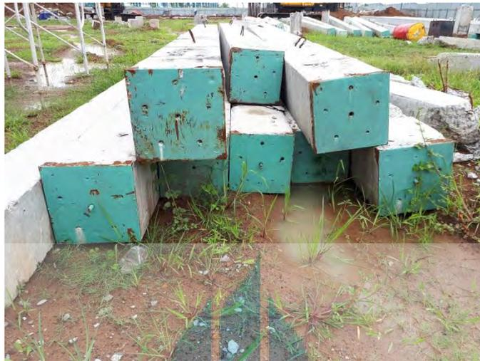
Gambar 5.1 Precast Reinforced Concrete Pile
