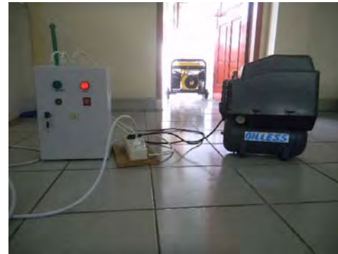
Figure 12. Photograph of ATS loading test using motor compressor 1.5 hp (1.1 kW), electricity supplied from PLN network
