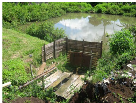
Figure 1.3. A simple toilet
