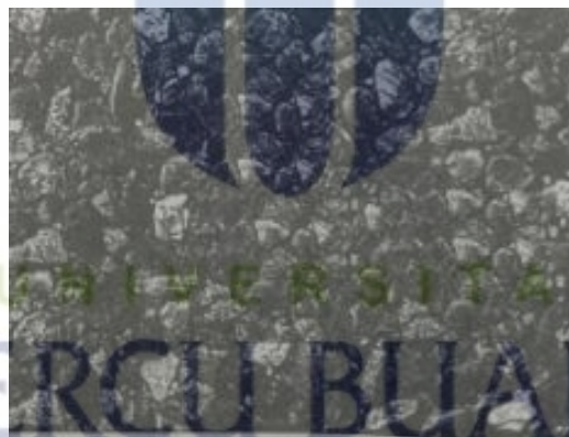
Gambar 2. 12 Kerusakan Pengausan Agregat ( Polished Aggregate )
