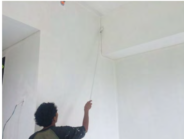
Gambar 4-5 Proses pengecatan dinding
