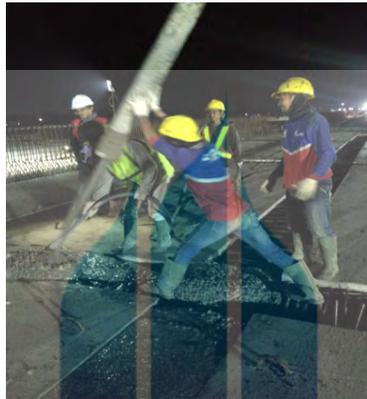
Gambar 4.3. Beton Ready Mix
