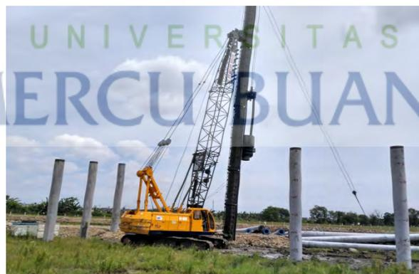
**Gambar 4.6. Diesel Hammer**
