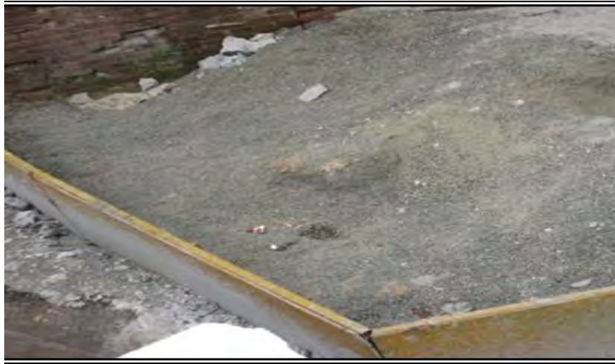
Gambar 4.2 - Pasir (Agregat Halus) Sumber : Proyek, 2018
