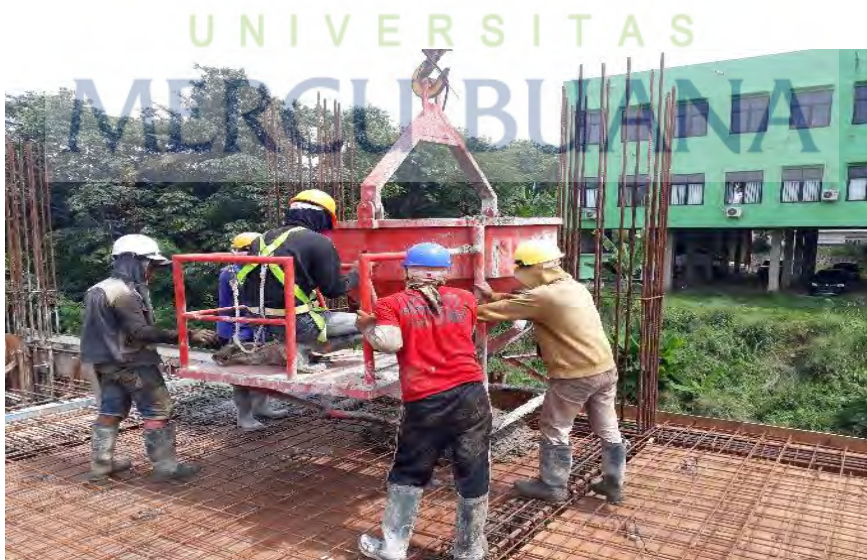
Gambar 4.14 - Concrete Bucket Sumber : Proyek, 2018
