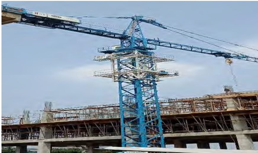
Gambar 4.8 – Tower Crane Sumber : Proyek, 2018
