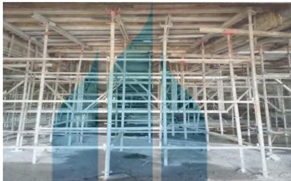
**Gambar 2. 1 Bekisting *Ring-lock***
