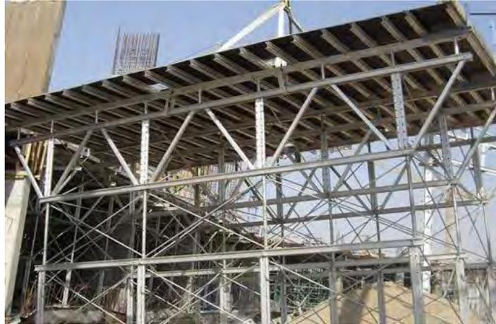
**Gambar 2. 3 Bekisting Aluma System**
