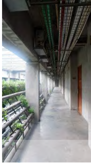
Gambar 2.23 Koridor Kamar Greenhost Butique Hotel
