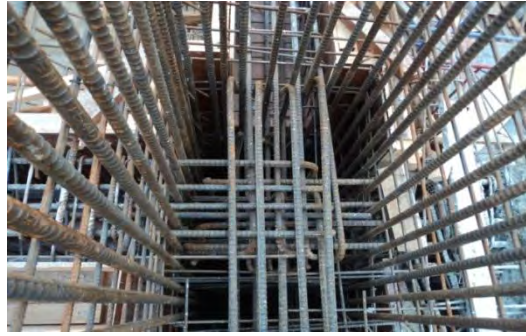
Gambar 5. 19 Beam & column joint
