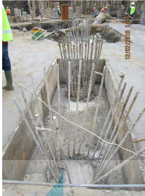
Gambar 5. 5 Pile Cap Tertanam
