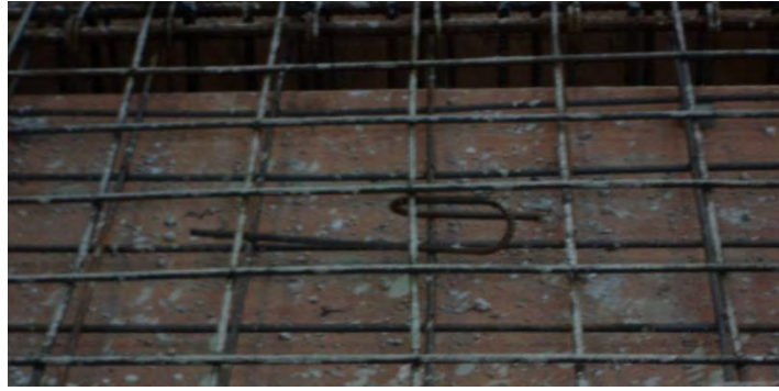
Gambar 5. 22 Decking besi plat lantai
