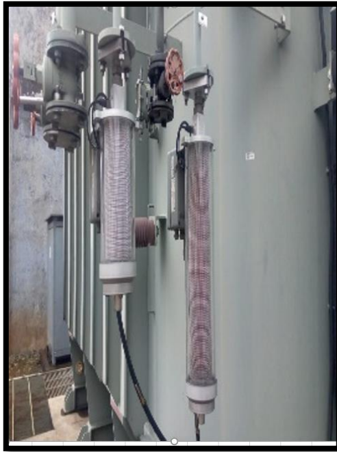
Gambar 2.6 Dehydrating Breather
