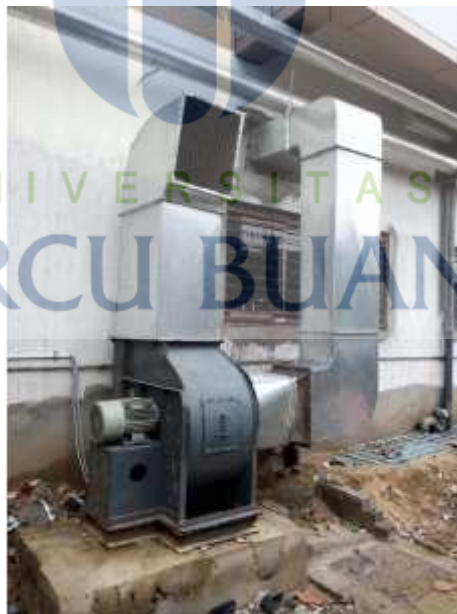
Gambar 2.6. Fresh Air Ducting
