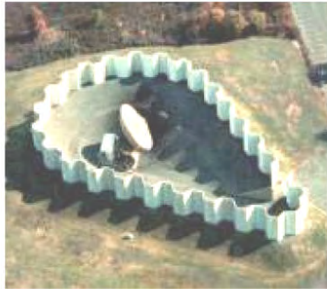
Gambar 3.29 Optimised shielding screen di AS
