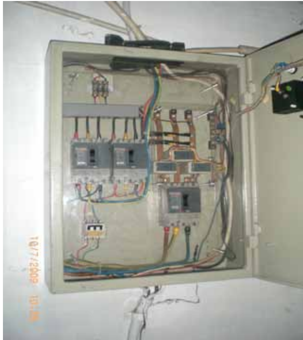
Gambar 6.20 Panel power ac central L4G1
