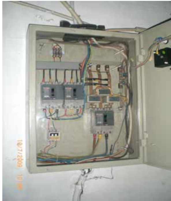
Gambar 6.22 Panel power ac central L6G1
