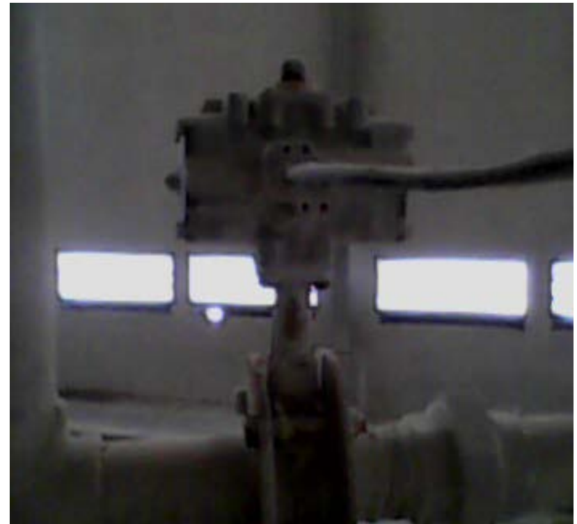
Diagfrahm Valve SIRAI L182-NPT 1 inch, 2/2 NC, pilot operated
