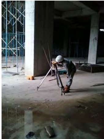
Gambar 5.16 pengukuran as/grid
