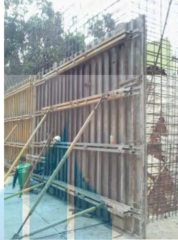
Gambar 5.18 bekisting retaining wall
