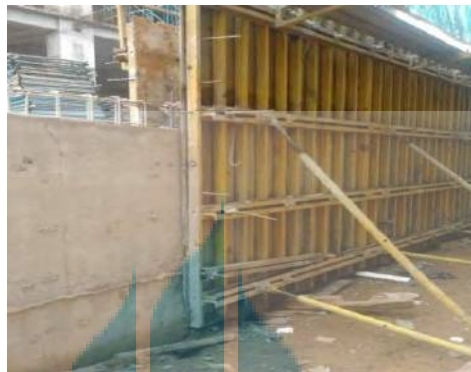
Gambar 5.19 pembongkaran bekisting retaining wall
