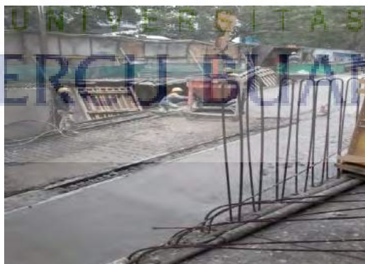
Gambar 5.42 pengecoran ramp
