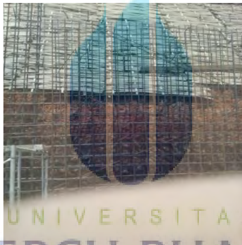
Gambar 5.15 pembesian retaining wall
