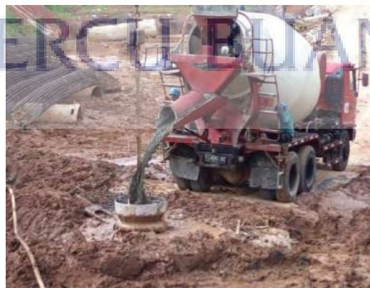
Gambar 5.7 pengecoran pondasi bored pile
