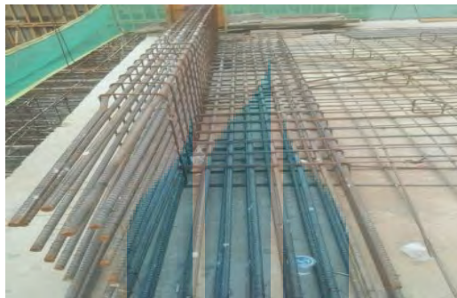
Gambar 5.32 pembesian core wall
