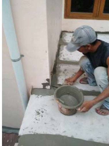
Gambar 2. 14 Pekerjaan Grouting Panel Lantai
